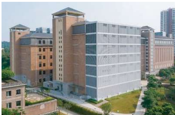
Ping An Guanlan No.3 Data Center
