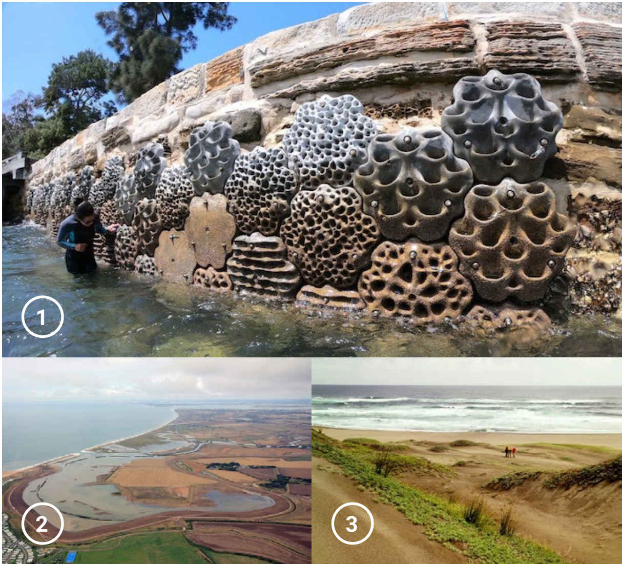
Figure 1: Examples of NbS projects worldwide; (A) The Living Seawall project in Australia’s Sydney Harbour, (B) the Medmerry scheme for coastal realignment, Sussex, UK, (C) construction of hybrid dunes in Barcelona for urban coastal defence.
