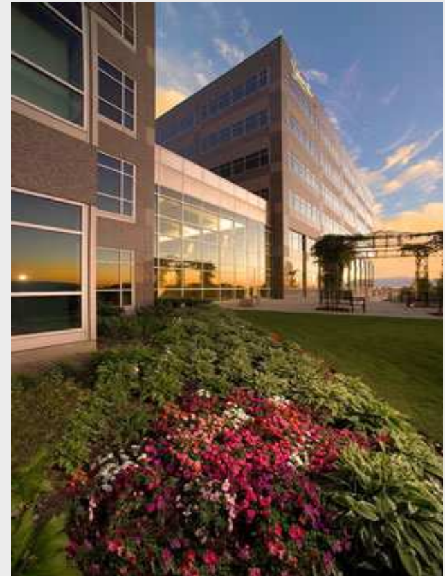
Cottonwood Corporate Center Salt Lake City, UT ENERGY STAR 2006-2009 BOMA TOBY Award 2009 Pursuing LEED Certification
